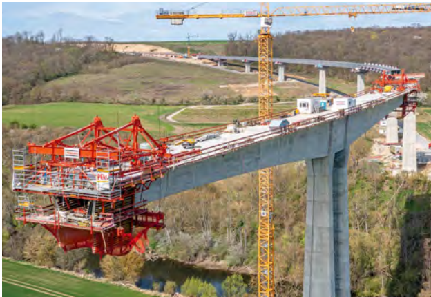
The Saaletal Bridge was built using a hybrid construction method. For the section that was implemented using the balanced cantilever construction method, the VARIOKIT VBC Balanced Cantilever Carriage was used for the first time in Germany.
