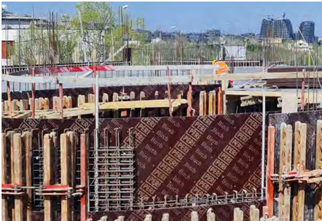
PERI Formwork Systems featuring PERI Birch Formwork Panels played a decisive role in the construction of the circular building sections.
