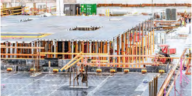
The PERI ALPHADECK formwork was used for 5,000 m² of formwork surface and impressed the customer in particular with its innovative drophead system for early stripping.
