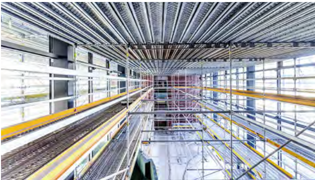
A special feature of the project is the lobby, which required the construction of almost 2,000 m 3 of scaffolding for its steel structure and suspended ceiling.
