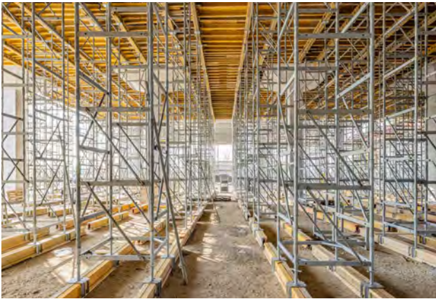
The use of PERI’s compatible formwork and shoring systems enabled smooth integration and efficient execution.
