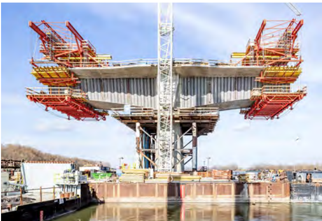
By using the VBC Formwork Carriages, it was possible to build the bridge efficiently using the cantilever construction method with a shorter construction time.
