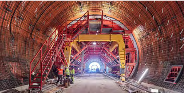
The customised formwork carriage from PERI offered the possibility of hydraulic movement with a pneumatic vibration system.
