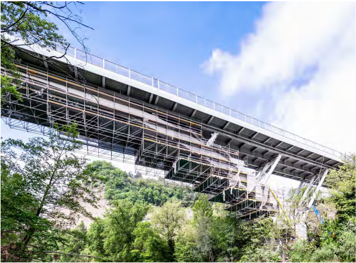
San Leonardo Bridge, Sasso Marconi, Italy
