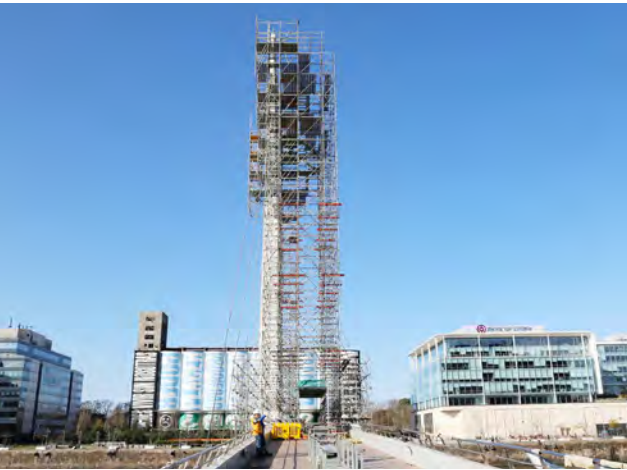
The scaffold used for renovating the mast of the Puente de la Mujer was 40-m high and solved the challenge posed by the low load limit of the pedestrian bridge.
