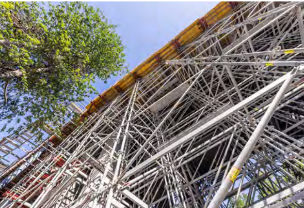
The combination of scaffolding, formwork and climbing systems made for a stable overall solution.
