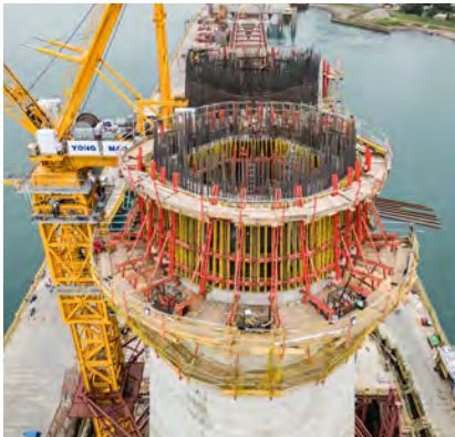
The two PERI SCS and ACS Climbing Systems facilitated quick, safe and efficient construction of the unique pylon structure.
