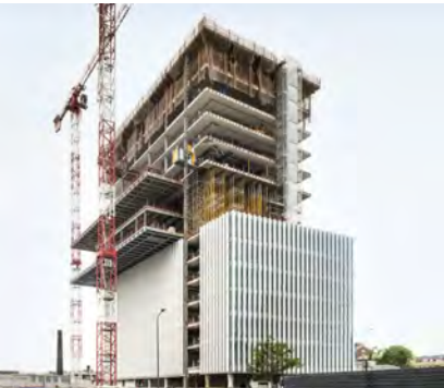
Three stacked yet offset structures are a special feature of the building, which were created with the aid of PERI Systems.
