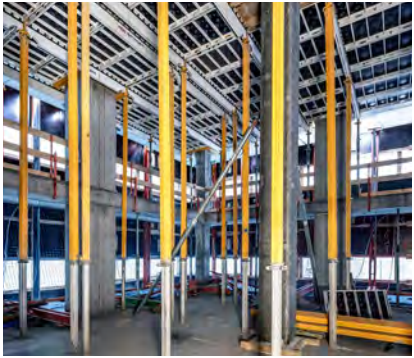
The lightweight, easily manageable system components of the SKYDECK Panel Slab Formwork enabled energy-saving work processes and short shuttering times.
