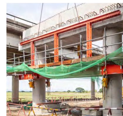
VPS paved the way for short concreting cycles and enabled the 250 cross girders to be completed on time.
