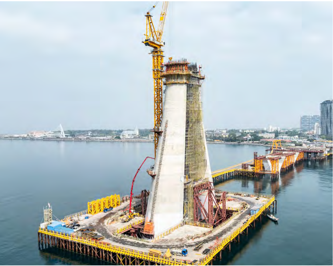
Danjiang Bridge, New Taipei, Taiwan
