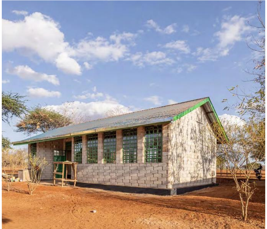
Second PERI School in Kitui, Kenya, built with TwistBlocks. More on the PERI Group's corporate citizenship: www.peri.com/sustainability
