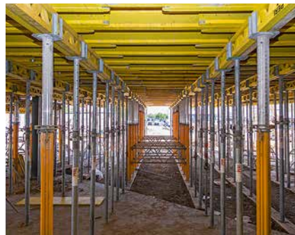
For applications with the GT 24, fewer girders, steel waling or slab props are required. This results in savings in both material and labour costs.
