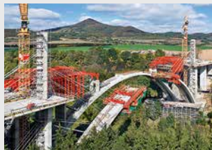
Bridge Formwork
