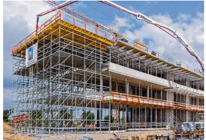
Complete solution from one source: wall and slab formwork as well as the shoring and reinforcement scaffolding were optimally adapted to match the project requirements.
