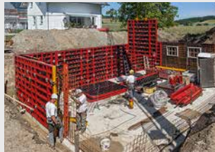
Wall Formwork
