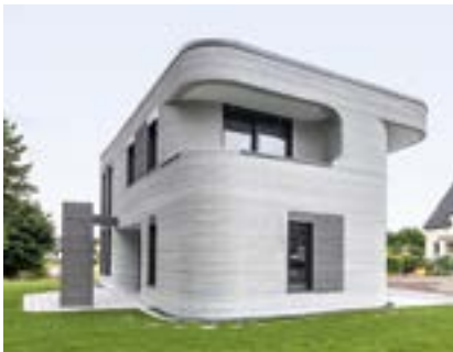
Germany's first 3D-printed residential building in Beckum with curved walls exemplifies the considerable design freedom offered by 3D construction printing.
