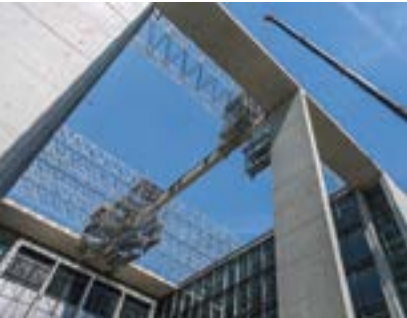
Even at great heights, working platforms of up to 20 m in length can be erected on the basis of the truss system.
