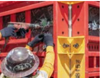
The InSite Construction Pressure Sensor is another building block for achieving an expedited concreting process.
