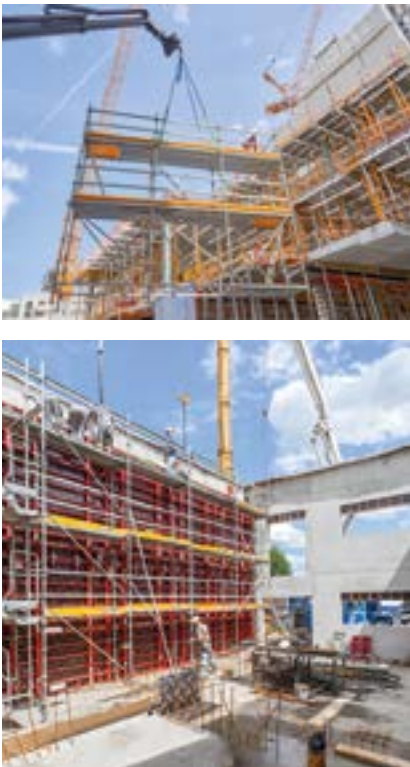
The PERI UP Reinforcement Scaffold can be used in front of formwork and walls without any ties or ballasting.
