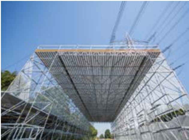
Bridging with spans of up to 8.50 m can be realised with the manageable system lattice girder. For example, this makes it possible to bridge uneven terrain or busy roads in a cost-effective manner.
