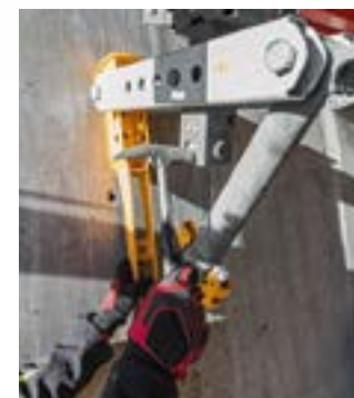
A hammer blow is all that is required to trigger the quick-release mechanism of the roller drop head. In the new cycle, it is simply brought back into the concreting position.
