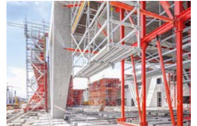
In combination with VARIOKIT, the PERI UP Scaffolding Kit allows safe access to various work areas.
