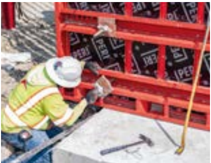
The innovative connection technology using X-Bolts and T-Bolts enables fast assembly and disassembly of the formwork.
