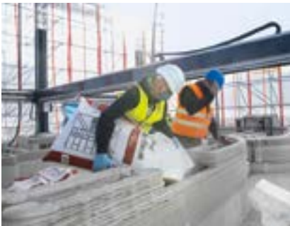
Integrating other trade activities into the printing process, such as insulation material or cable ducts, further increases efficiency.
