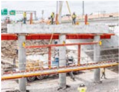
The innovative split-soffit striking method speeds up the cycle time enormously, meaning that fewer formwork sets are required.
