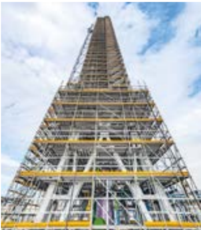
During use, the non-slip perforated decks, circumferential guardrails and yellow toe boards ensure a high degree of occupational safety.
