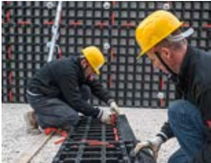
All accessories such as connectors and corner posts have been designed to be as versatile as possible. This reduces the material requirements on the construction site.
