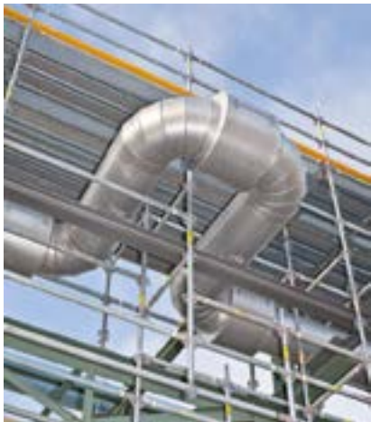
The self-locking ledger connection on the scaffolding node (Gravity Lock) and the integrated lift lock in the decks can speed up the assembly process.
