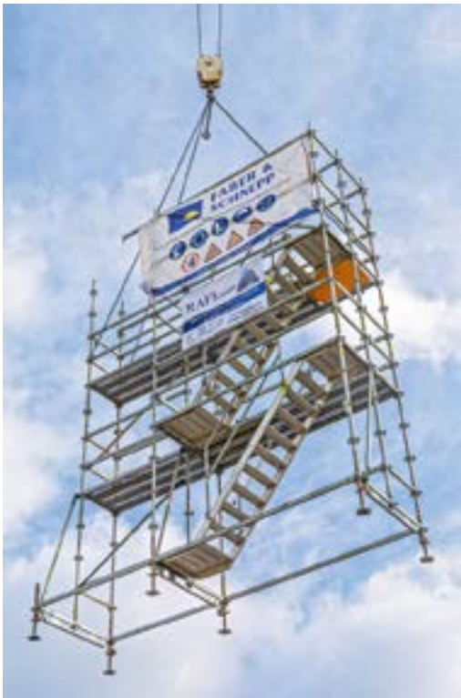
Thanks to pre-assembled units, the material requirement can be determined quickly, thereby facilitating the planning process.
