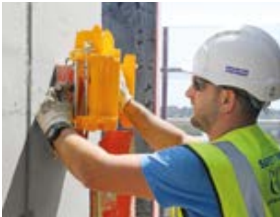
RCS MAX offers the user intuitive assembly with lightweight system components. In addition, the climbing shoes can be installed safely and conveniently without the need for a ladder.
