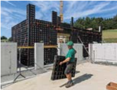
The low number of different system components means that assembly can be carried out quickly and easily, always following the same assembly logic.
