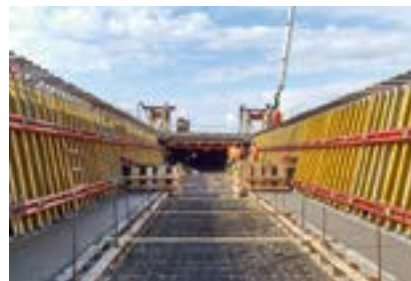
The flexible VARIOKIT formwork units can be individually adapted to suit the substructure and bridge geometry.
