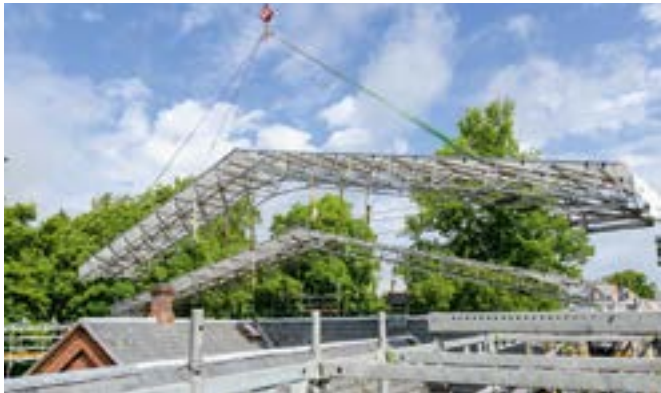
The PERI UP Weather Protection Roof can be erected independently of the substructure. Assembly is carried out without formwork girders and couplings.
