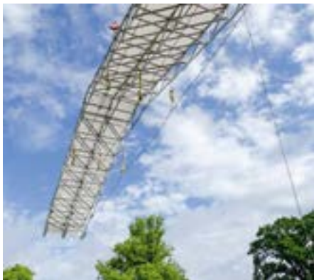
Pre-assembly of the truss units is carried out from a safe position on the ground. Lifting is done by crane.
