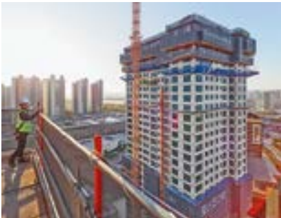
The synchronous climbing of all platforms increases safety on the construction site. Open building edges are thus a thing of the past. This eliminates tripping hazards and the risk of falling parts.
