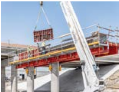
With VSS, the side formwork can be used independently. This means that the striking process can be carried out the following day and that the reinforcement work can be carried out conveniently.
