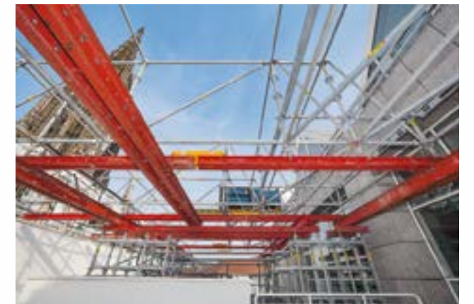
In case of limited space or an unstable substrate, VARIOKIT can also be used as a load-bearing base for various PERI UP scaffolding solutions.
