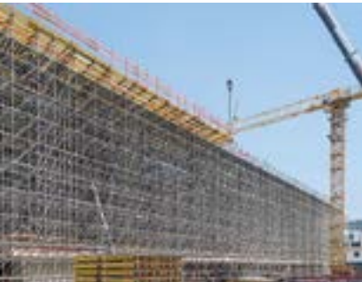
PERI UP Shoring Towers are compatible with PERI Slab Formwork Systems and are also designed for use with standard steel and timber construction dimensions.
