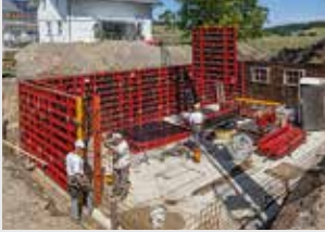
Wall Formwork
