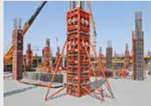
Column Formwork
