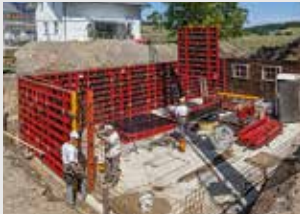
Wall Formwork
