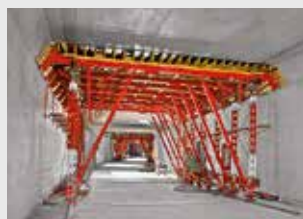
Tunnel Formwork
