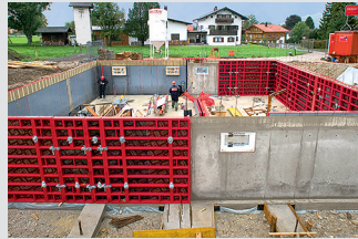
Wall Formwork
