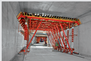
Tunnelformskalling
