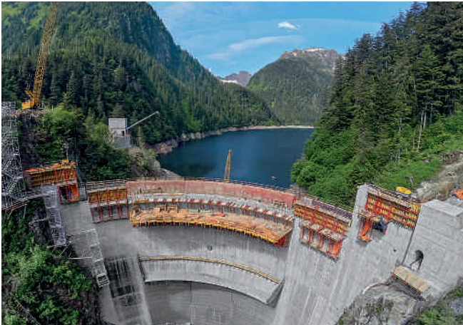
Dam upgrade project: as part of a hydroelectric power plant expansion in Alaska, the height of the dam wall was to be increased.
