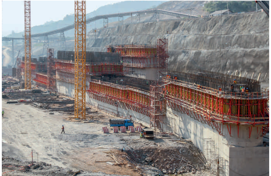
The high flexibility of the SCS Climbing System allowed an easy adaptation to suit all geometries in this dam project.
