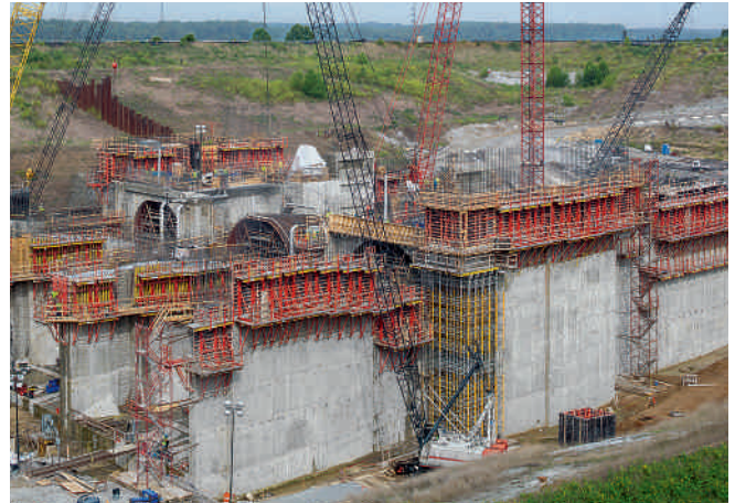
The massive power plant walls were single-sidedly formed and concreted using the SCS Climbing System.
