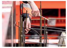
The installation of the ISC Thermocouples is very simple: Before the concreting process, you install them in the reinforcement.
