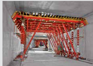
Tunnel Formwork
