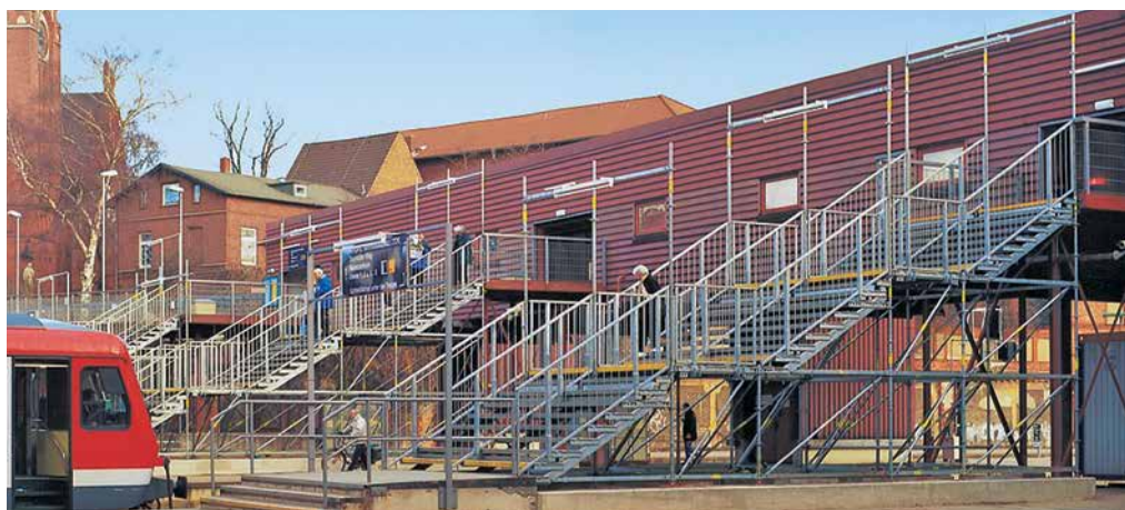
Entry to the railway platforms via temporary stairways and a temporary pedestrian bridge made it possible to separate the construction site for the new accesses of public traffic to the platforms.
