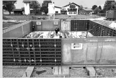
Wall Formwork
