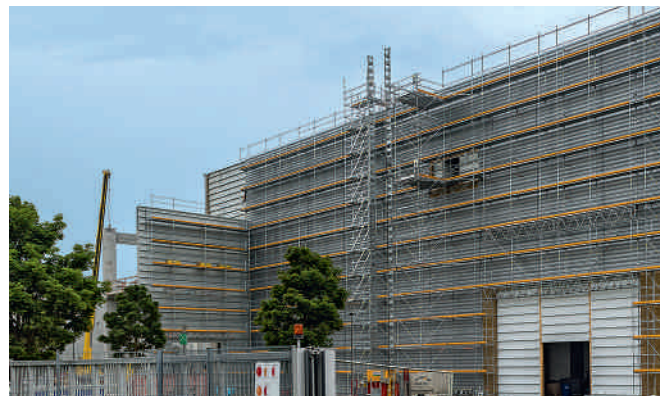
Expansion of the Zeiss Semiconductor Technology Plant, Oberkochen, Germany
