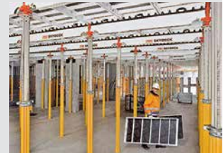
Slab Formwork
