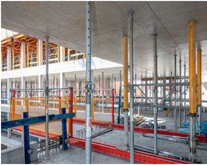
The RCS Rails of the RCS MP Landing Platform are clamped between two floor slabs by means of MULTIPROP Props.
