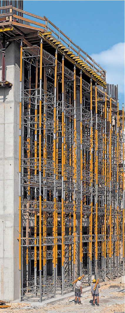
MULTIPROP Shoring Towers for scaffolding a 20 m high, cantilevered structural slab.
