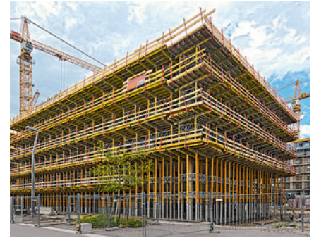
The PERI solution with MULTIPROP and MULTIFLEX, as well as for forming the circumferential balconies, served simultaneously as working scaffold.
