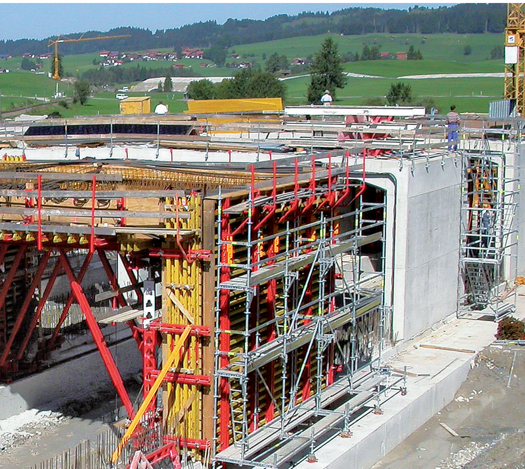
The combination of proven systems such as VARIO GT 24 and HD 200 with new elements from RCS or the diagonal strut, results in a cost-effective formwork carriage.
