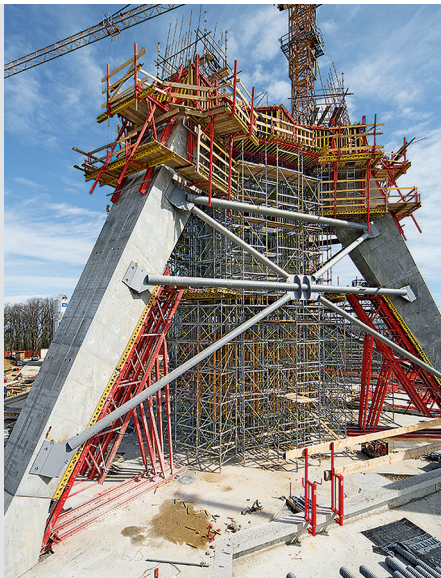
Same system components for providing temporary support for the structure as well as for climbing scaffold application.
