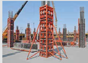
Column Formwork
