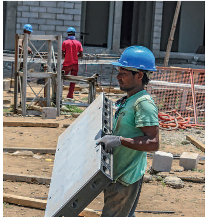
Fast shuttering and striking in India.
