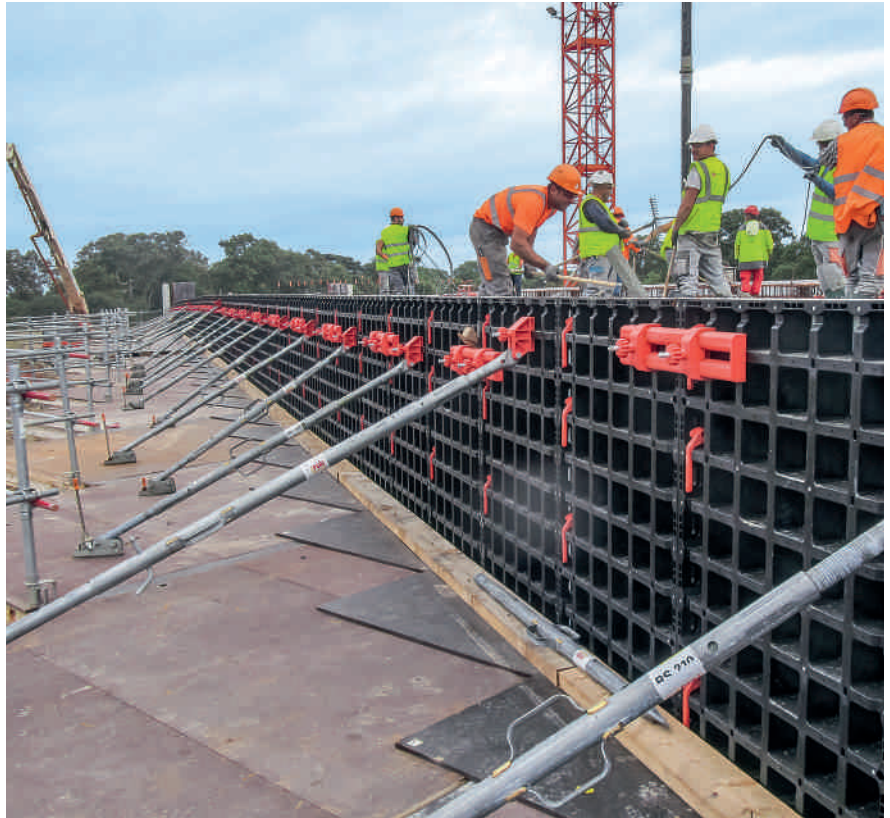
With small panel sizes and easy handling, DUO is predestined for the forming of foundations.
