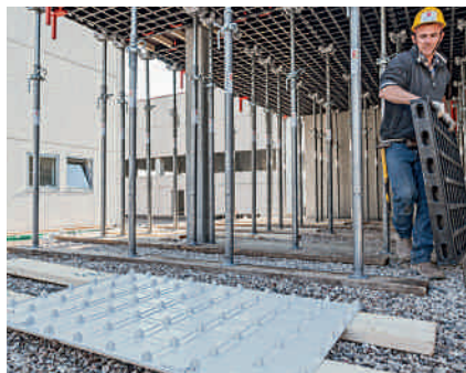
3. Pre-positioning the new formlining
