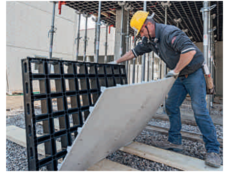
2. Removing the damaged formlining
