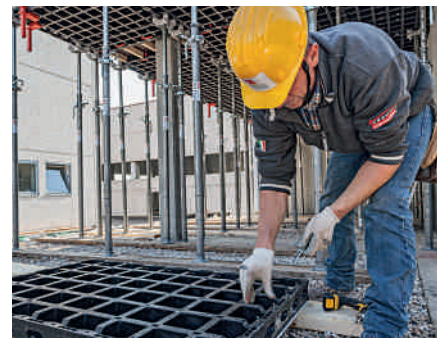
4. Screwing on the new formlining
