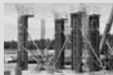
Column Formwork
