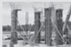
Column Formwork
