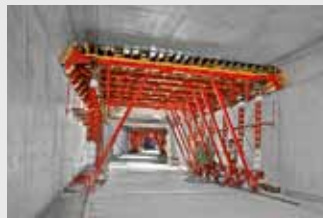
Tunnelformskalling
