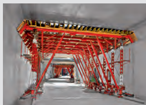
Tunnelformskalling
