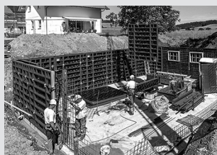
Wall formwork
