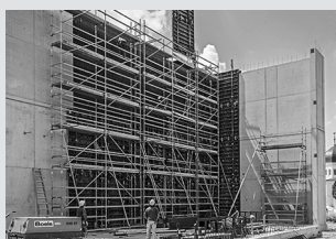
Working scaffold construction
