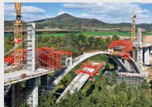
Bridge Formwork
